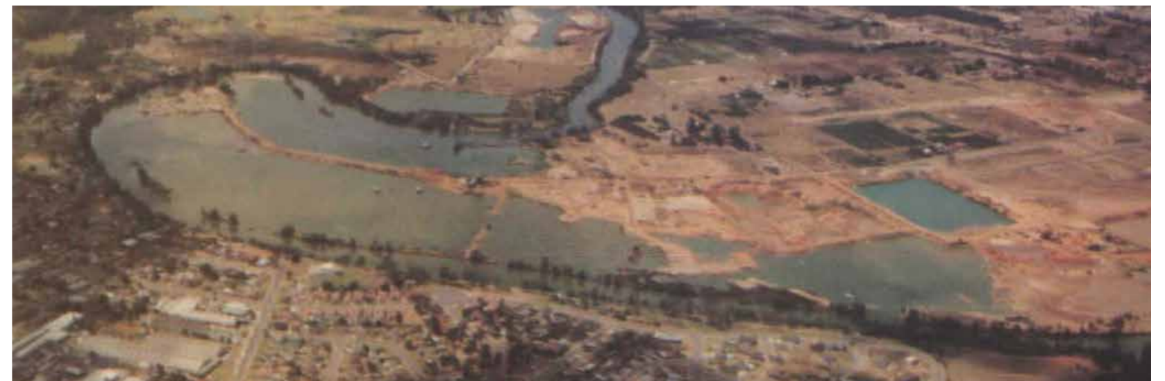
Sand Mining at Chipping Norton - January 1975
