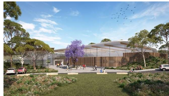
Draft concept designs from the Carnes Hill Aquatic and Leisure Centre MasterPlan
