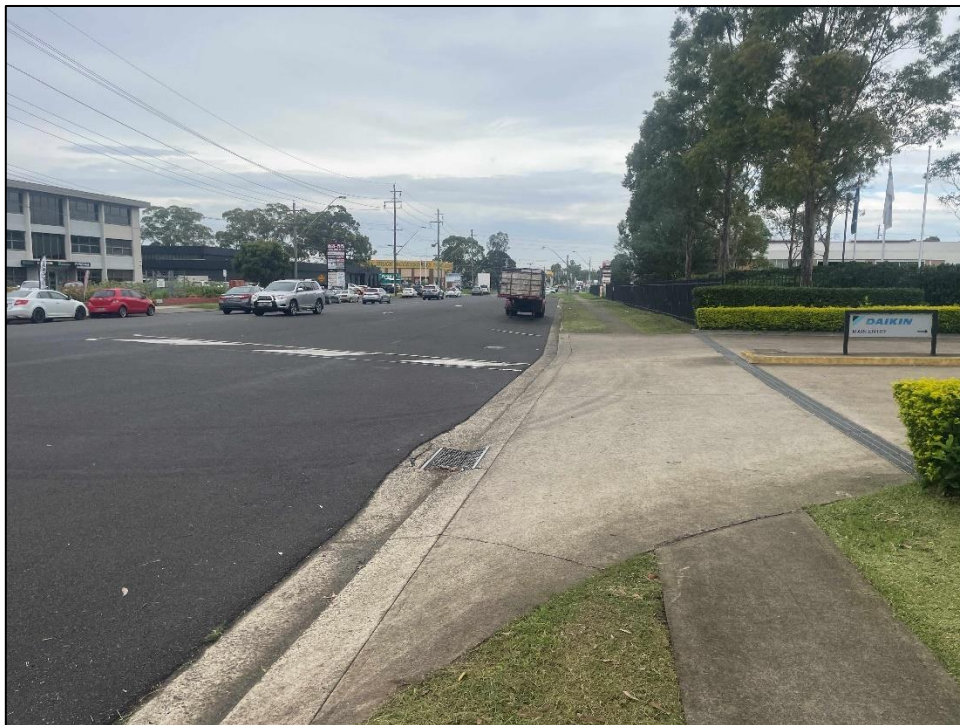
Above: Governor Macquarie Drive looking south
