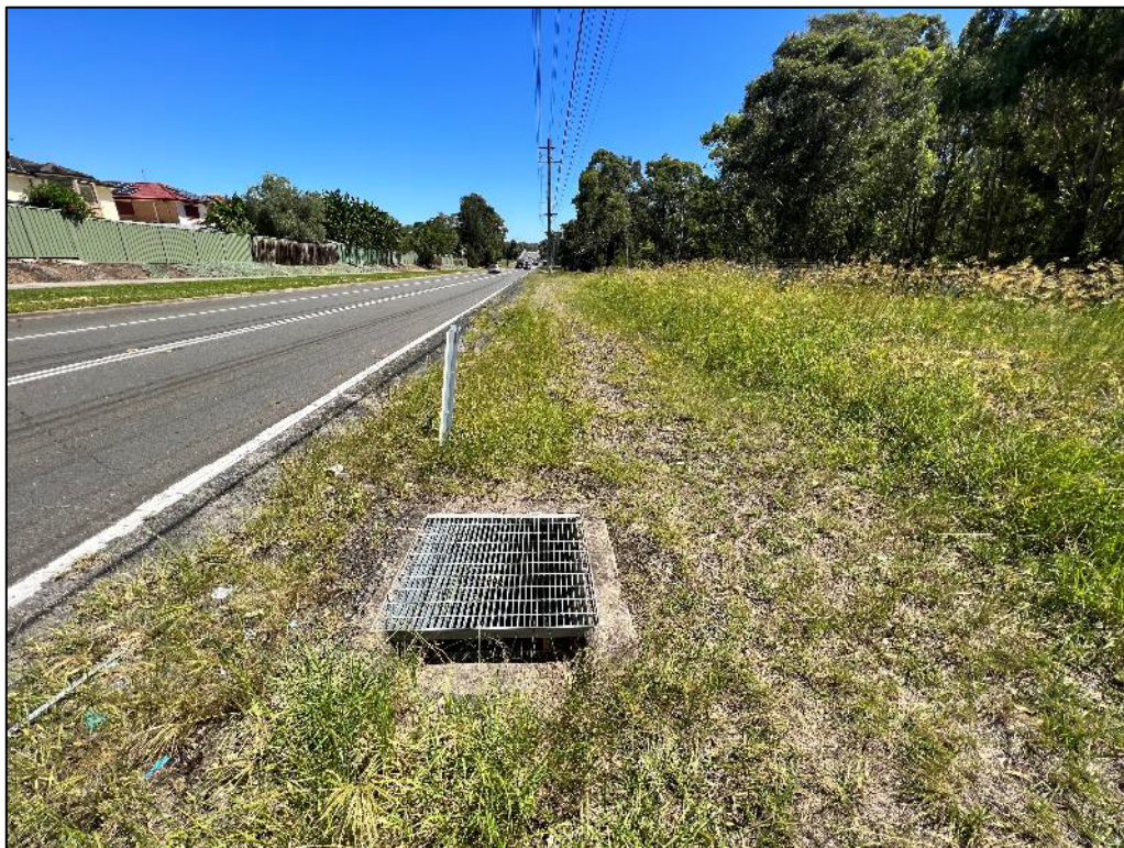
Plate 7: Looking west along the northern road verge of Kurrajong Road.
