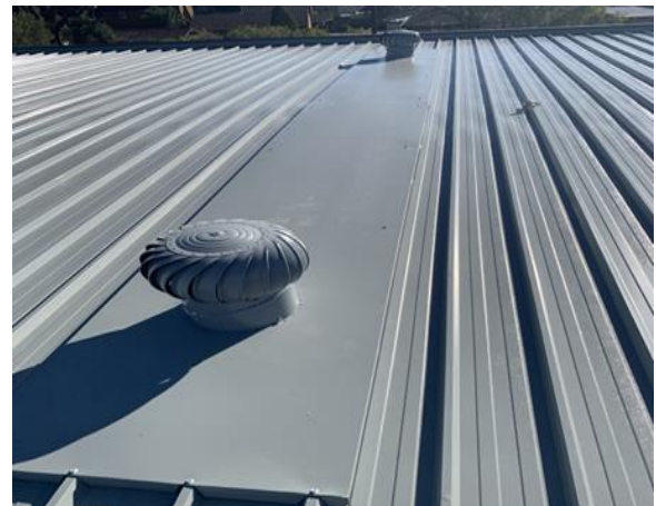
New roof - Frank Oliveri Community Hall
