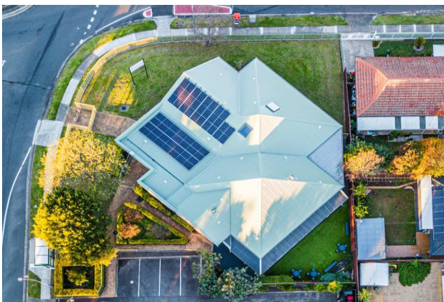
New Solar Panel - Hinchinbrook Community Centre
