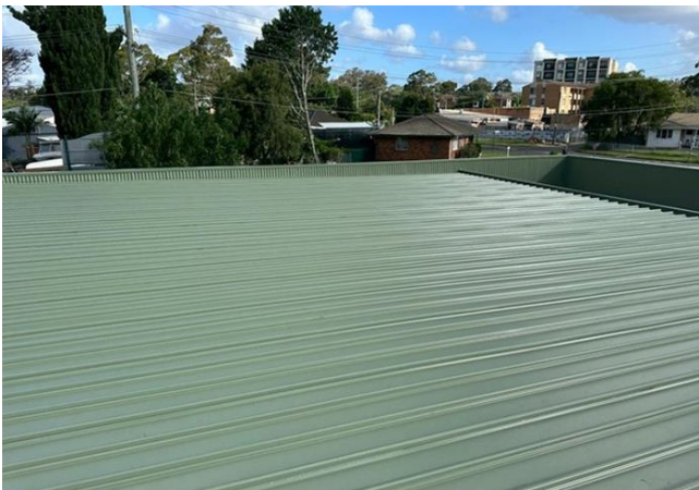
New roof - Warwick Farm Community Centre
