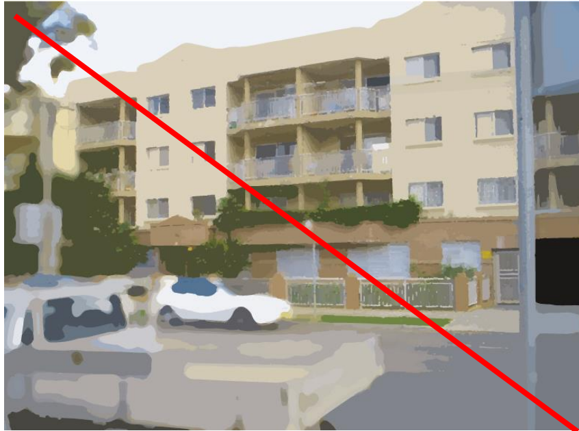
Figure 12 Car parking at ground level
