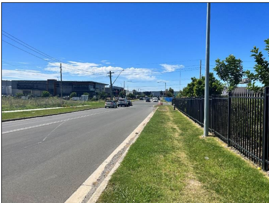
Plate 2: Looking east along the southern road verge of Yarrunga Street.
