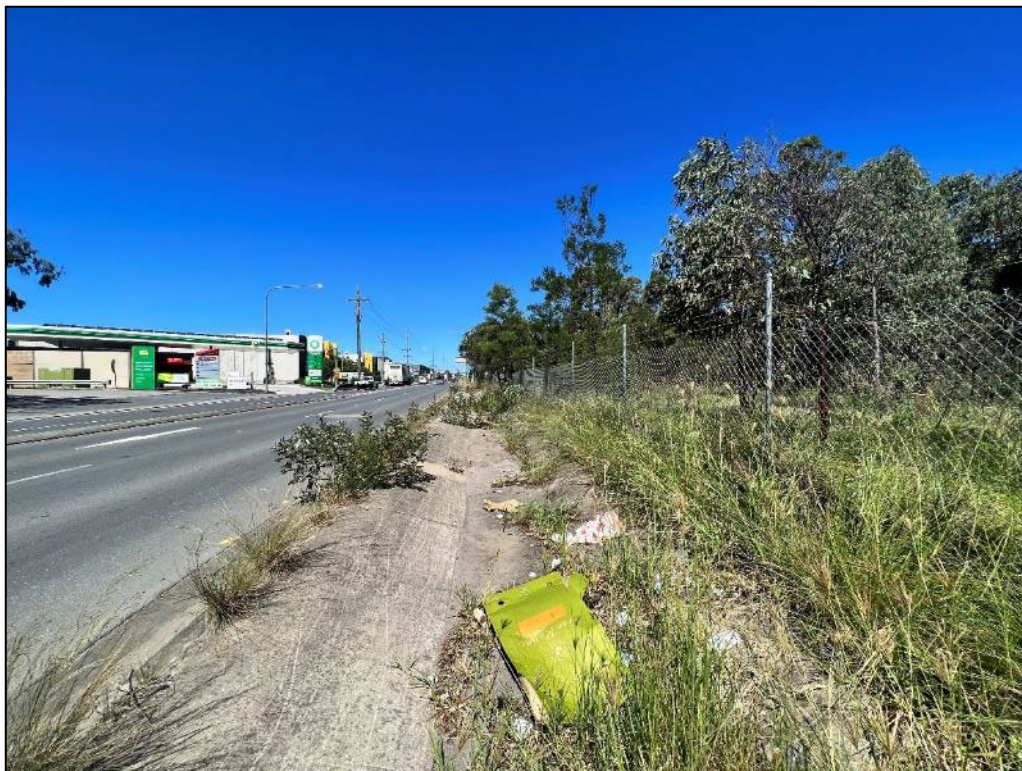
Plate 7: Looking south from the northern end of the Bernera Road upgrade section.
