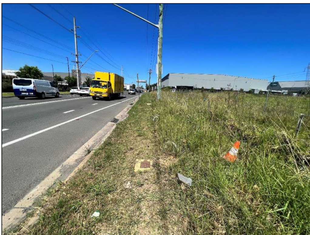
Plate 8: Looking south along the western road verge of Bernera Road towards the intersection upgrade area.
