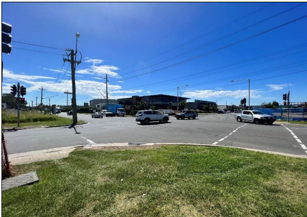
Plate 1: Looking north east across the proposed intersection upgrade area.
