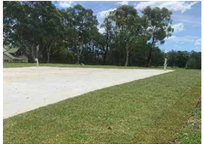
After – Concrete Works at Grand Flaneur Beach
