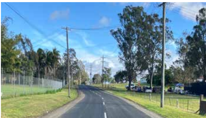
Road reconstruction – Gurner Avenue, Austral
