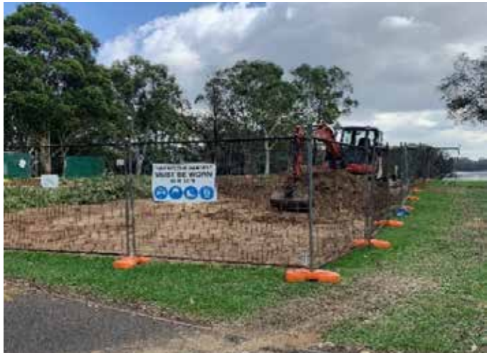
Before – Concrete Works at Grand Flaneur Beach
