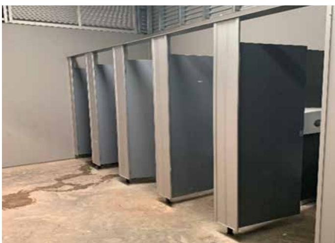
Before – Amenity upgrade at Ash Road
