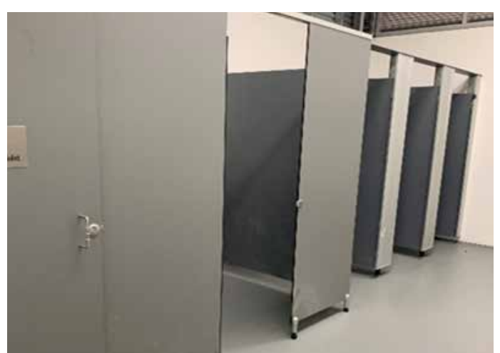
After – Amenity upgrade at Ash Road
