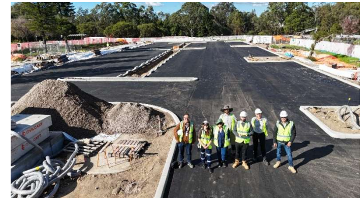
Stage 2 construction works at Light Horse Park
