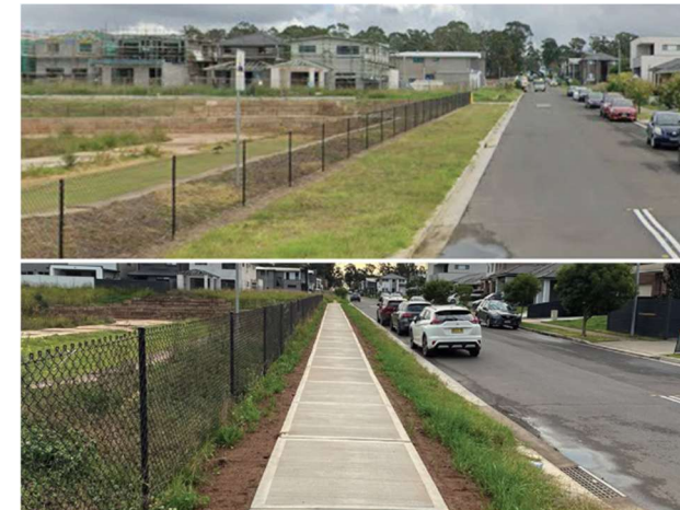
Footpath installation on Haybale Street, Austral
