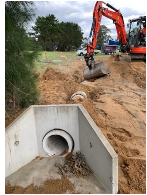
Stormwater pipe repair Grand Flaneur Beach, Chipping Norton.
