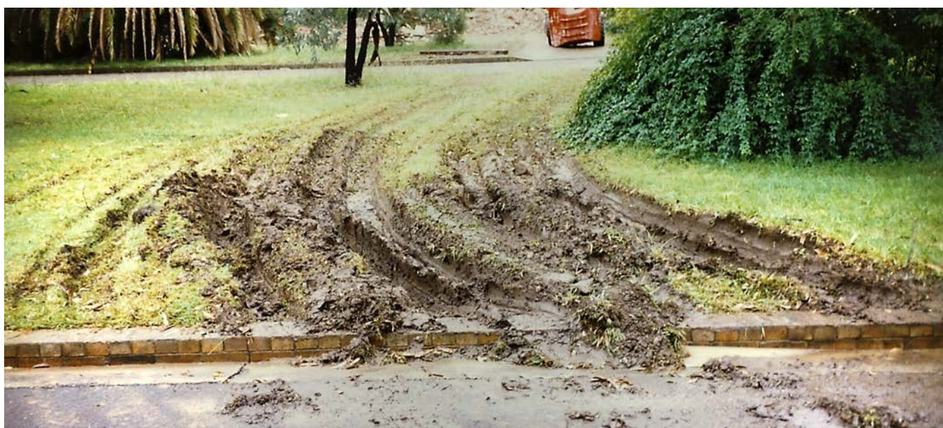
Figure 31: Trafficking of wet ground near to trees can have devastating effects to soil and roots and must be avoided. Temporary ground protection will normally be needed whenever vehicles need to cross soft ground to load and unload equipment. (Source: Arterra)
