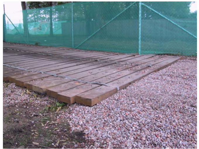
Figure 28: When access is required close to trees it may be necessary to install temporary or permanent ground protection to prevent root damage and soil compaction. (Source: Arterra)
