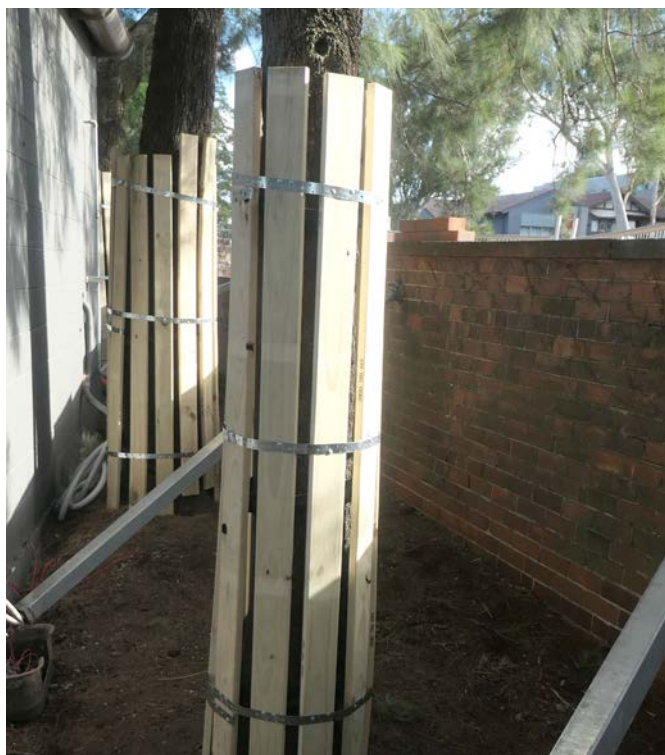
Figure 26: When working close to trees, it may even be necessary to install temporary trunk protection measures to limit accidental damage to delicate bark and branches. (Source: Arterra)
