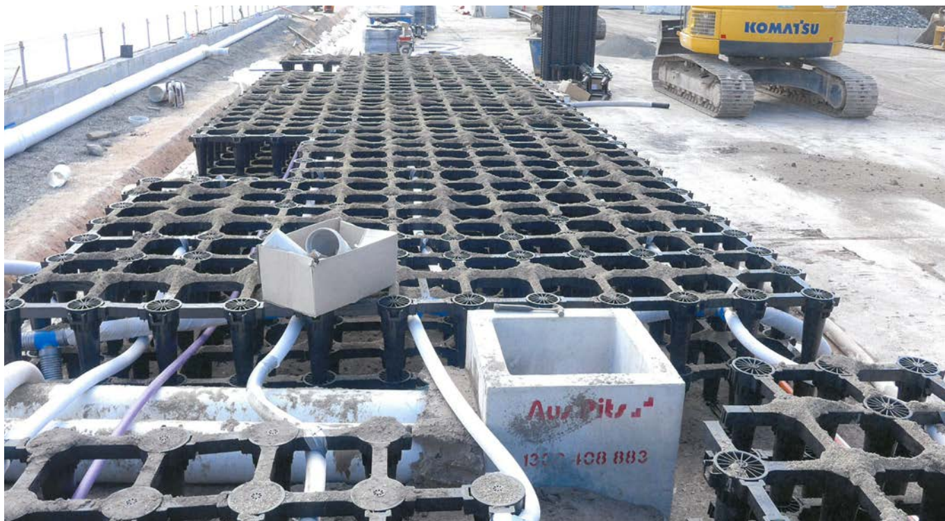
Figure 56: Numerous methods are now available for integrating trees and their necessary soil volumes within urban environments while still allowing pavements and roads to continue successfully above. The above illustrates a proprietary system, Strata Vault by Citygreen, being used at Barangaroo Sydney. (Source: Citygreen)
