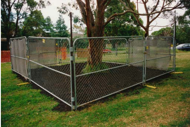
Figure 27: A key protection measure is the provision of adequate exclusion fencing to protect both the above and below ground portions of the tree from damage. (Source: Arterra)
