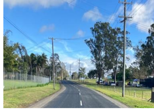
Road reconstruction - Gurner Avenue, Austral.
