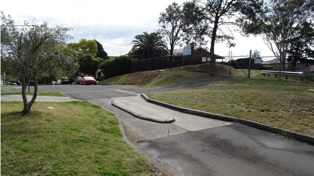
Figure 5 Bus filter outside 22 Box Road, Casula
