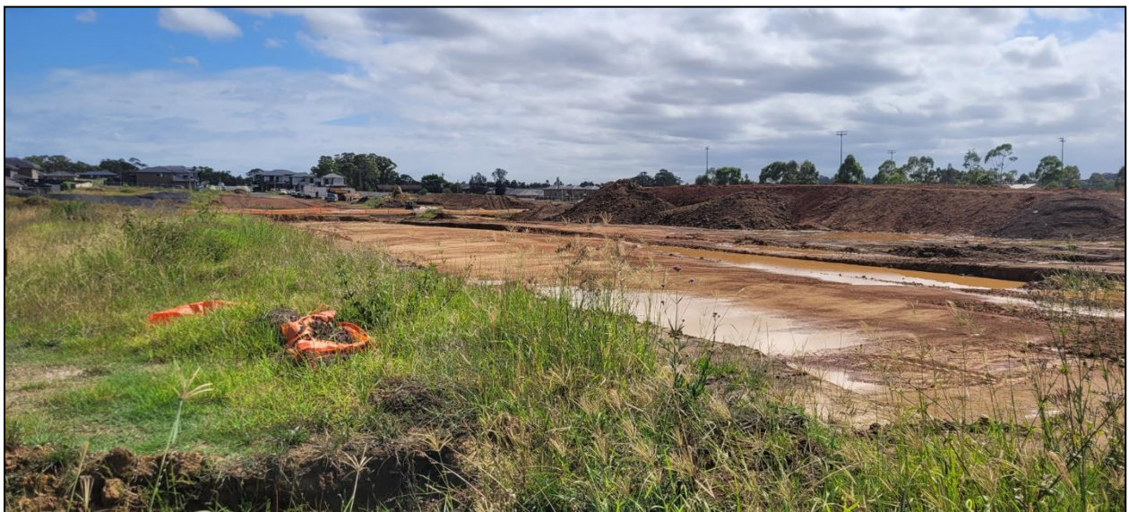
Figure 5 – View of drainage work from Hall Circuit
