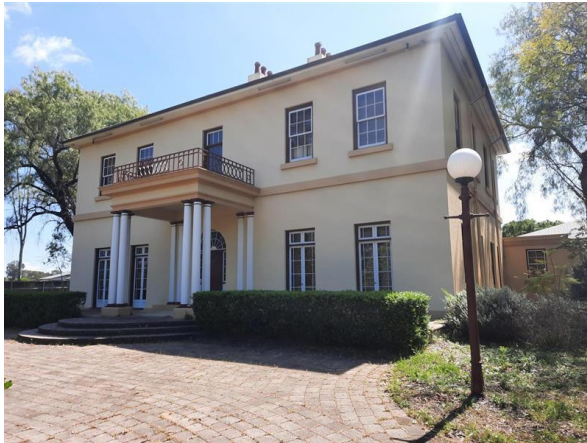
Figure 6: Southern view of existing homestead
