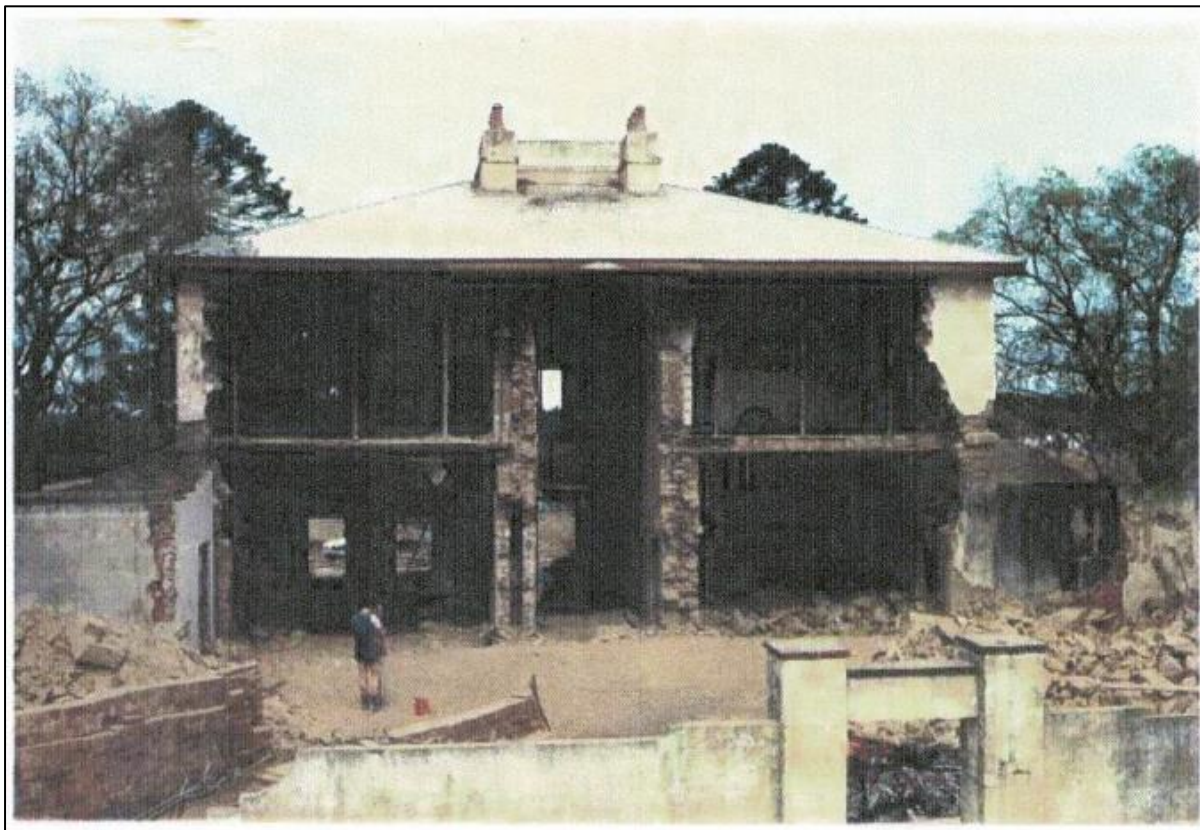
Figure 18: Partially demolished Horningsea House 1982
