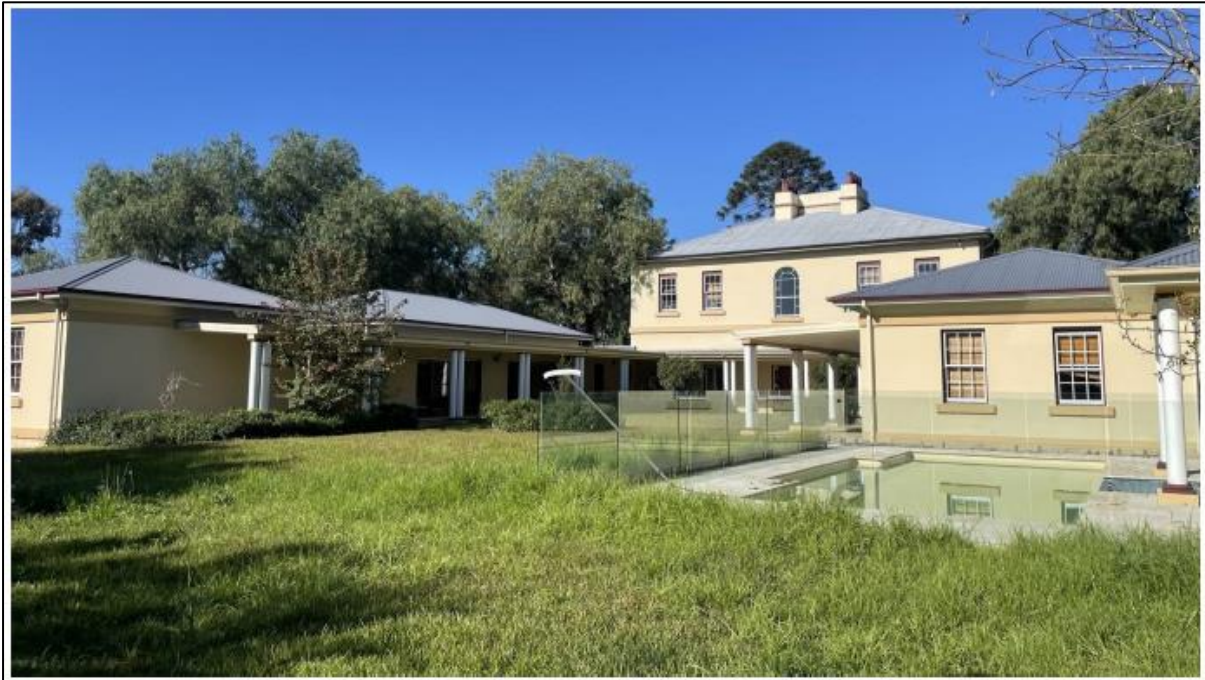
Figure 20: Rear of the property 2024.
