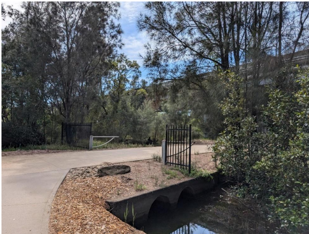
Figure 11 – Existing pathway at the southern boundary of the proposed works area leading to the M5 Motorway (source: Patch)
