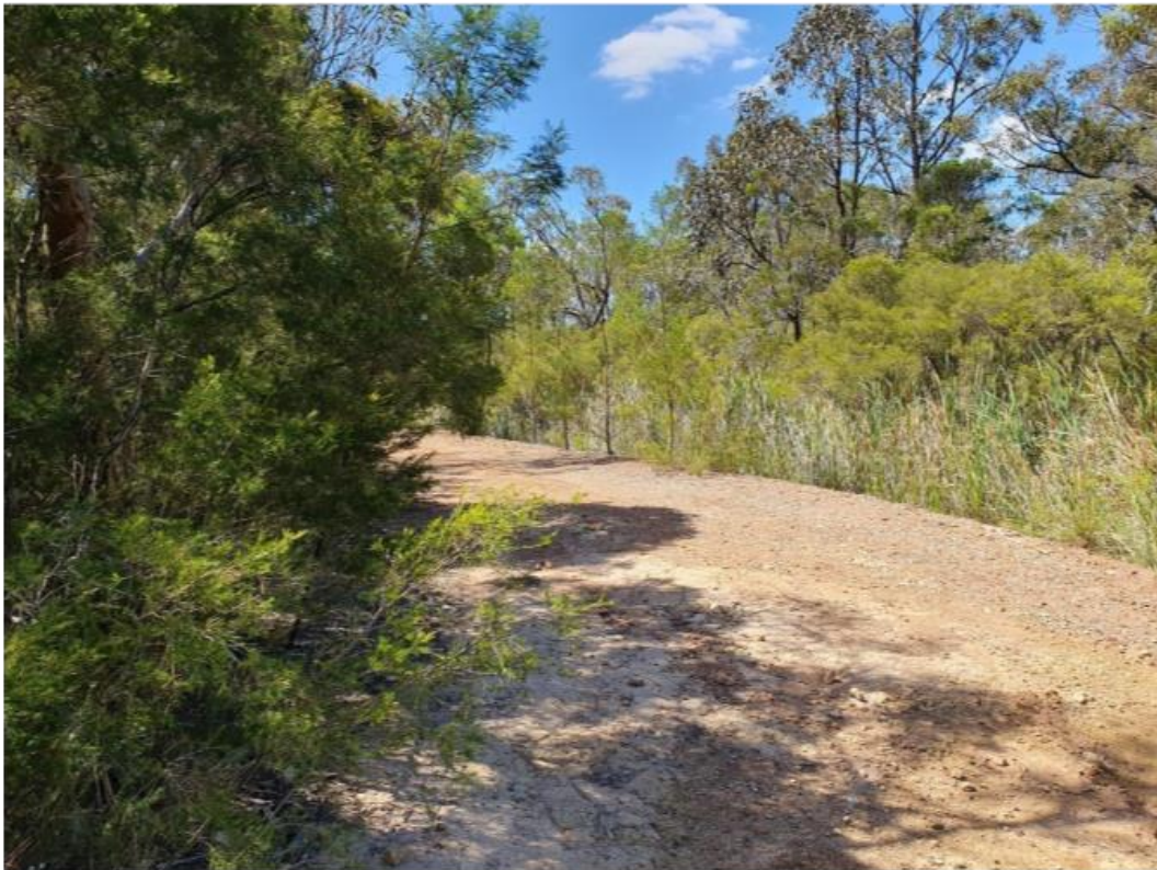
Figure 5 - The existing fire trail in the west to east directed section of Stage 1 of the proposed development
