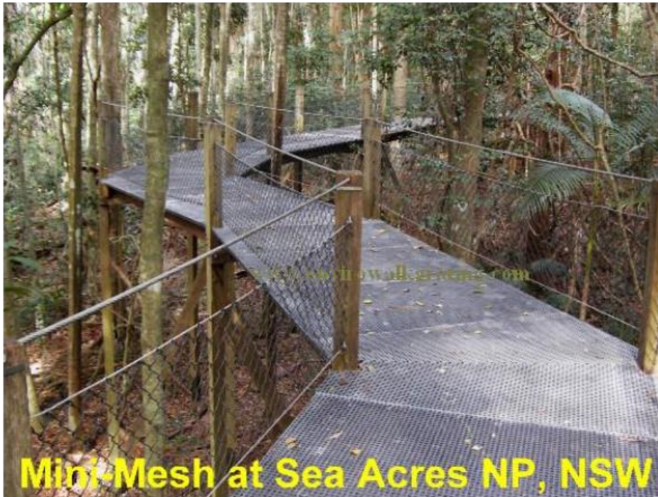
Figure 20 - Example boardwalk construction that would be used winding through individuals of trees that would be used in the current proposal
