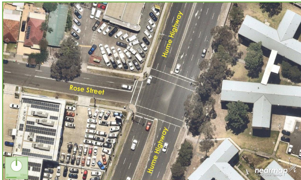
Figure 5: Hume Highway and Rose Street
