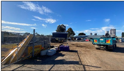
Photo 3. Rose Street Depot, taken from the rear boundary, looking north-east.
