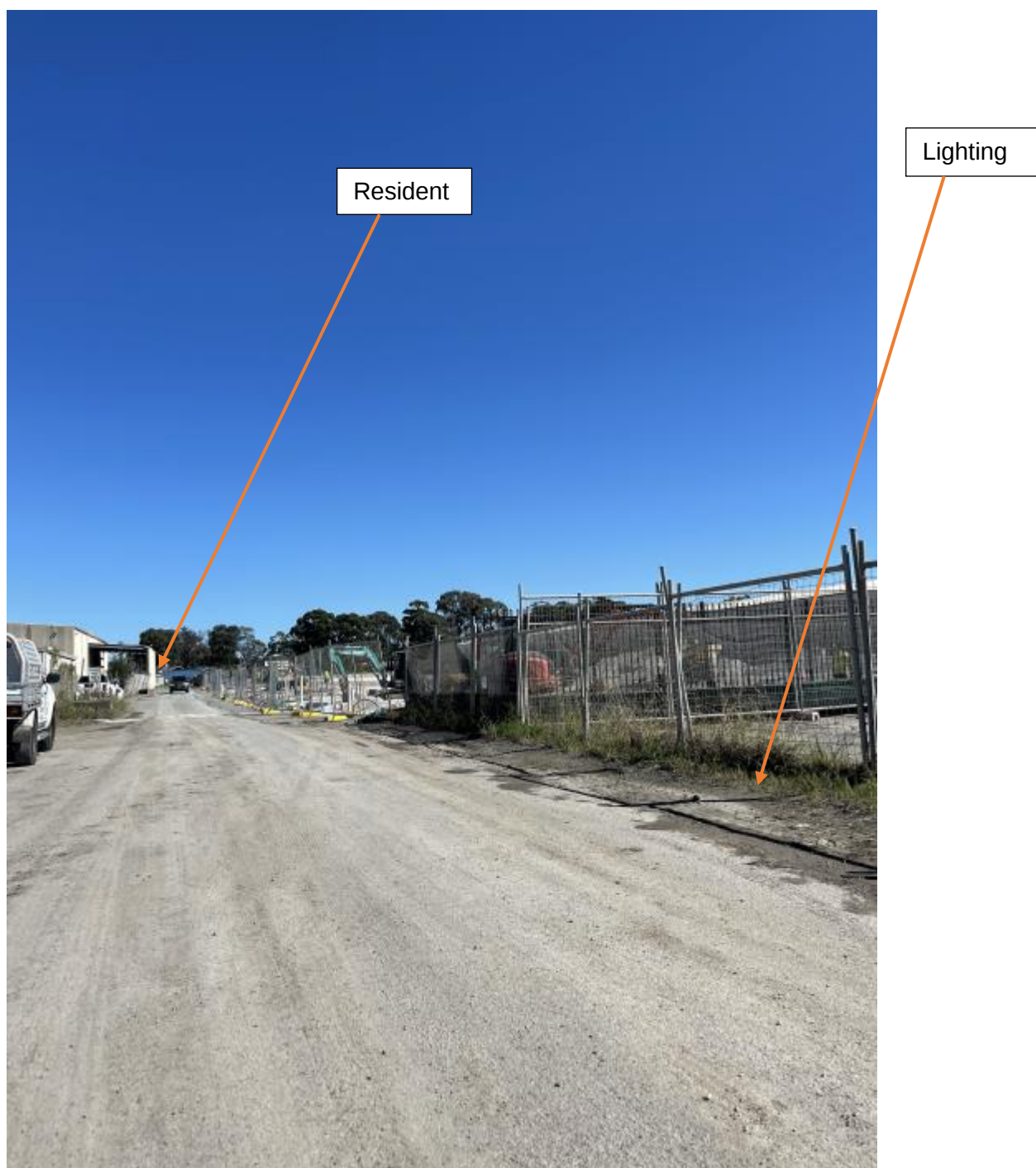
Figure 8: Site Inspection (Location of proposed lighting on site) (Note: Image shows distance for proposed lighting on site appropriately setback from residents)
