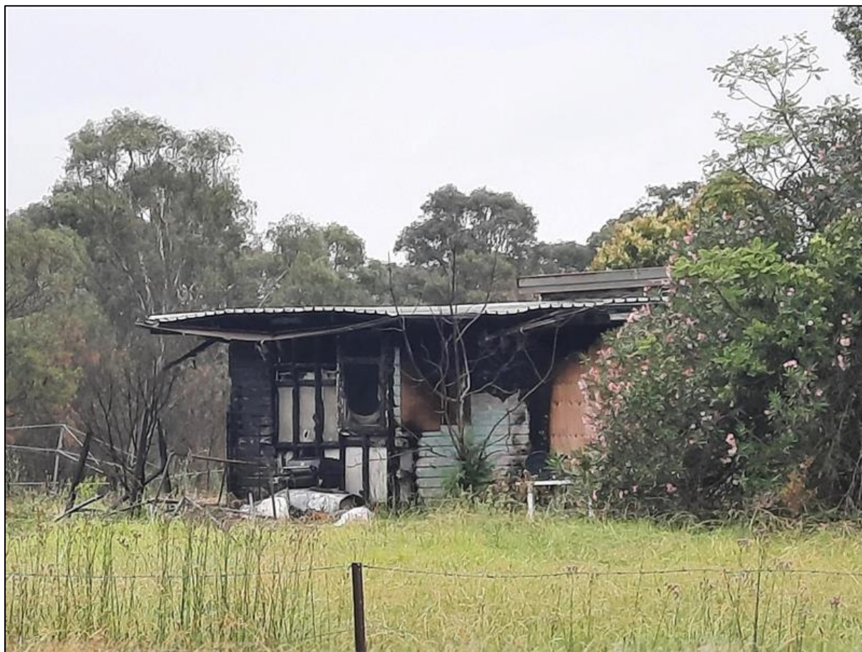
Figure 6: Subject site - current condition (18 December 2024)
