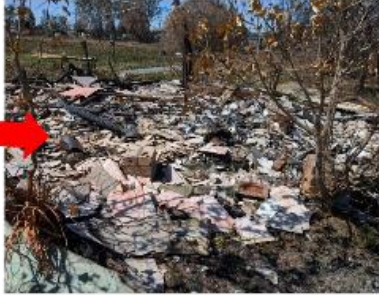
7. Fire damage to structures south of the house. Extensive asbestos debris present.
