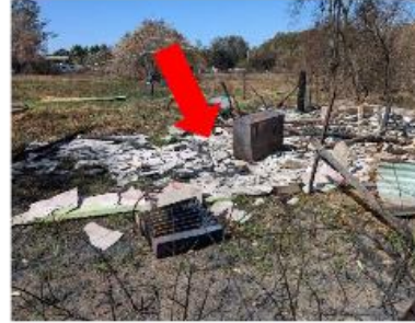
8. Fire damage to structures south of the house. Extensive asbestos debris present.
