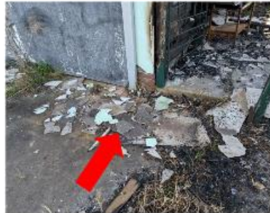
4. External, south of house, debris below damaged eaves - fibre cement sheet
