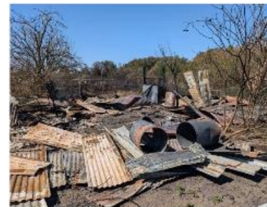
4. External, south of house, debris below damaged eaves - fibre cement sheet
