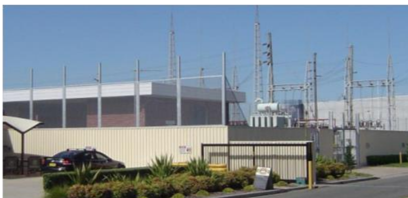
Endeavour Energy's Seven Hills Zone Substation is an 'outdoor' design. Note height of fencing due to adjacent 'climb point' created by the seating and awning.
