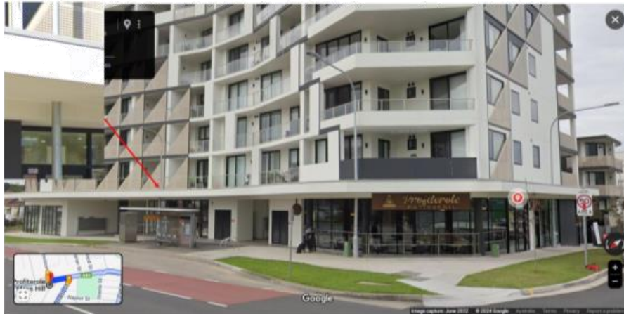
The street awning is inappropriately constructed around three streetlight columns. Source: Google Maps Street View.
