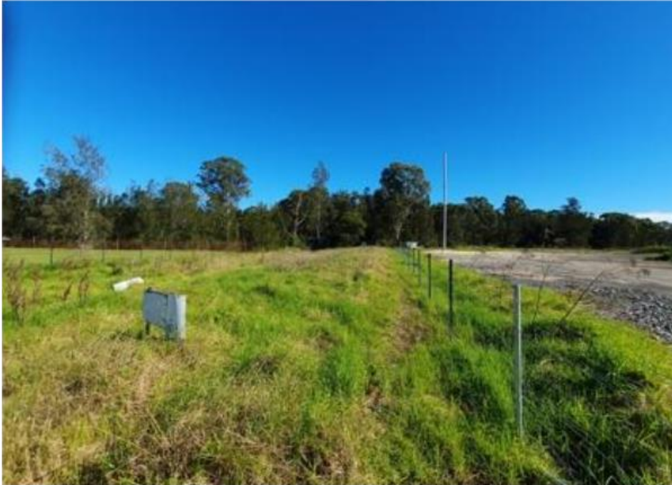
Figure 7 View looking towards Bonds Creek from the bottom of Eleventh Ave showing location of new stormwater pipes with subject site on the right
