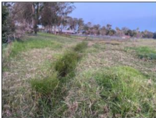
Figure 3.4 View northeast across the northern section of the project area showing an excavated drainage channel
