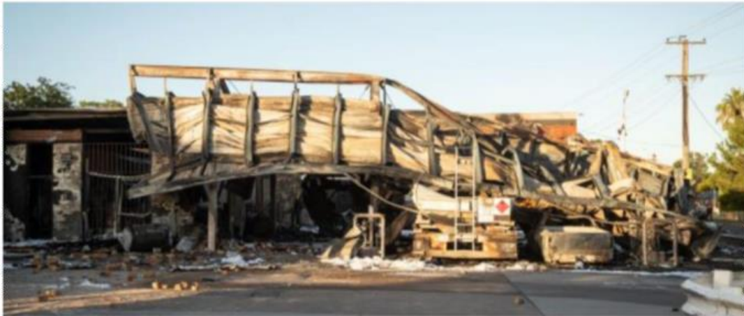
Figure 4: Service Station Facility Following Fire
