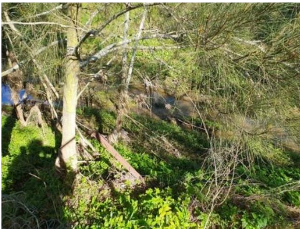
Figure 10 View from the top of levee at outlet site 2 showing weedy ground cover of
