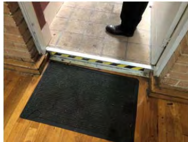
Image 5: Trip hazards evident at junction of doorways to sports hall. In particular the entry to amenities (pictured) and store room.
