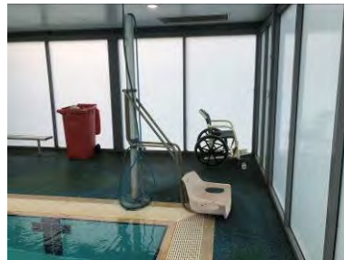
Image 5: A disability hoist – in wrong location
