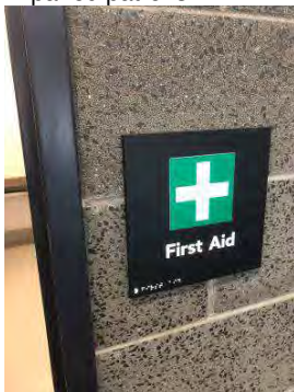
Image 4: All signage is DDA compliant including tactile braille indicators and clearly defined symbols and contrast for visual impaired patrons.
