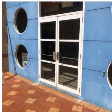
Image 2: Several of the door thresholds require a ramp, so to mitigate the existing step and potential trip hazard.
