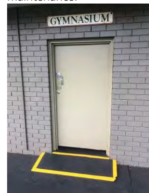
Image 9: Entry to fitness room not appealing, and door threshold (ramp) may be DDA compliant
