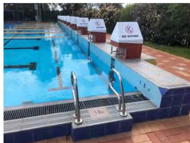
Image 8: Pool climb outs acceptable and step from pool concourse to pool edge is acceptable – however height to starting blocks is not.
