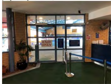
Image 5: Entry to aquatic area is restrictive via single entry door only. No airlock.
