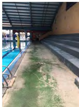
Image 8: Pool concourse in need of repair along 25m pool and tiered concrete seating
