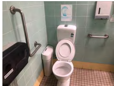
Image 2: Tiled floor in good condition. Accessible pan should be installed with a back rest.
