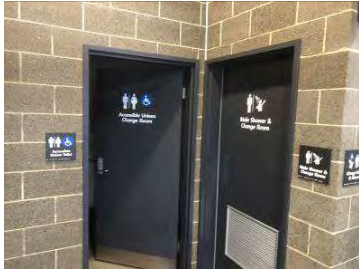
Image 1: All signage is DDA compliant including tactile braille indicators and clearly defined symbols and contrast for visual impaired patrons.
