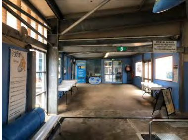
Image 1: Link building to main entry / reception. No air handling system evident. This may be causing the 'thermal - cold bridging effect' and condensation to glazed surfaces.
