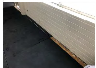
Image 6: floor matting to be repaired at edges. Requires general maintenance.
