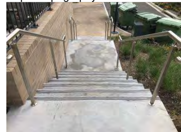
Image 6: External stairs not DDA compliant as ground tactile indicators are not installed.
