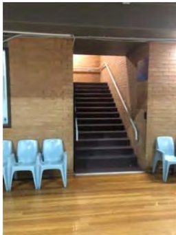
Image 4: Handrails are not compliant as they don't extend 300mm past the top and bottom riser.
