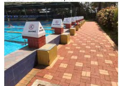
Image 9: Starting blocks to be removed to make way for removable ones. Depth of pool to be confirmed if acceptable for competition diving.
