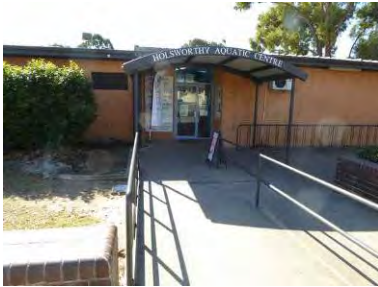
Image 1: Handrails at entry are not AS 1428 / BCA complaint (however may not be required for access)
