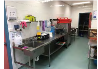
Image 3: Wash area in good condition. Dishwasher should connect to a mechanical exhaust system so to collect the steam.
