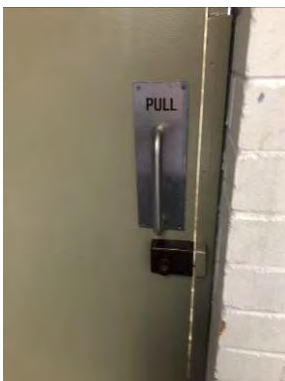
Image 7: Door handle and door lock not complaint to BCA. Door can be locked externally and not allow direct egress from room.
