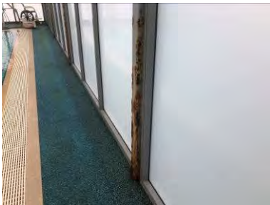
Image 4: Columns cast into floor are corroding
