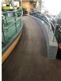
Image 5: Internal ramp to café level not to DDA / BCA code compliance and ground tactile indicators
