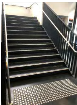
Image 4: All stair ways are fully DDA/ AS 1428 compliant.
