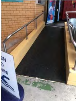
Image 4: Pool side ramp to café level not to DDA / BCA code compliance and ground tactile indicators
