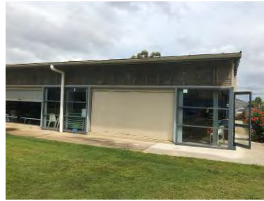
Image 8: mixture of tilt up / roller doors to façade of pool hall.
