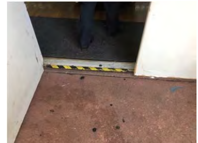
Image 6: Trip hazards evident at junction of doorways to sports hall. In particular the entry to amenities and store room (pictured).
