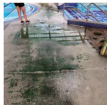
Image 12: Pool concourse in need of repair. Evidence of water pooling and poor surface drainage.
