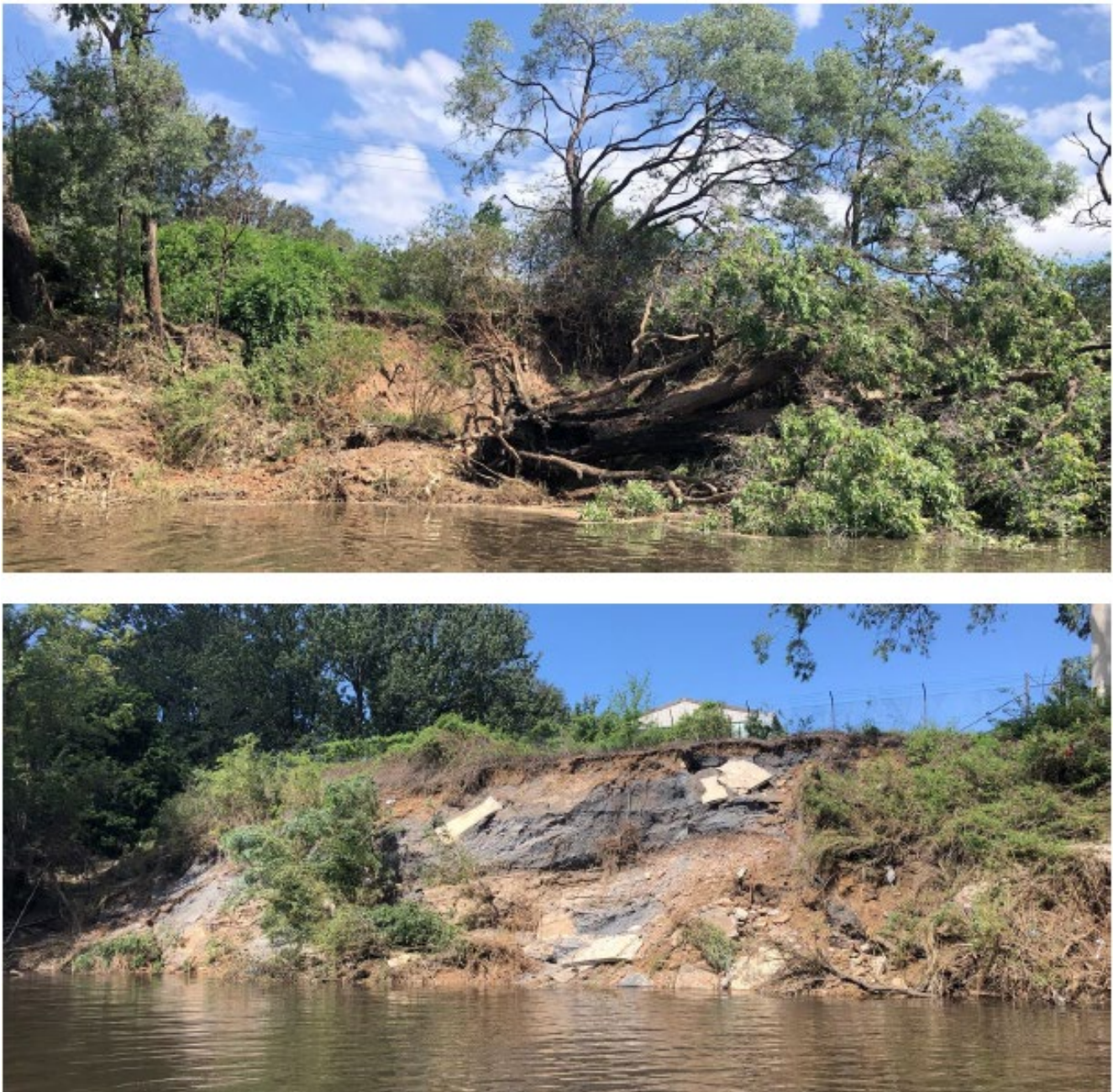
Figure 73: Bank Erosion at Moore Point February 2020
