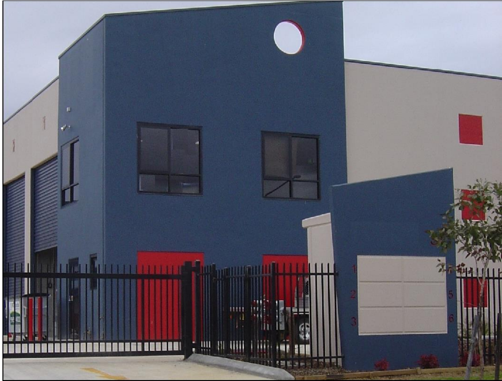
Figure 3 Character of Industrial Buildings
