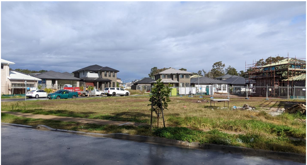
Figure 4 – Alternate view of the site (not all vacant land is part of the site) and recently/under constructed dwellings on Threlkald Avenue in the background.
