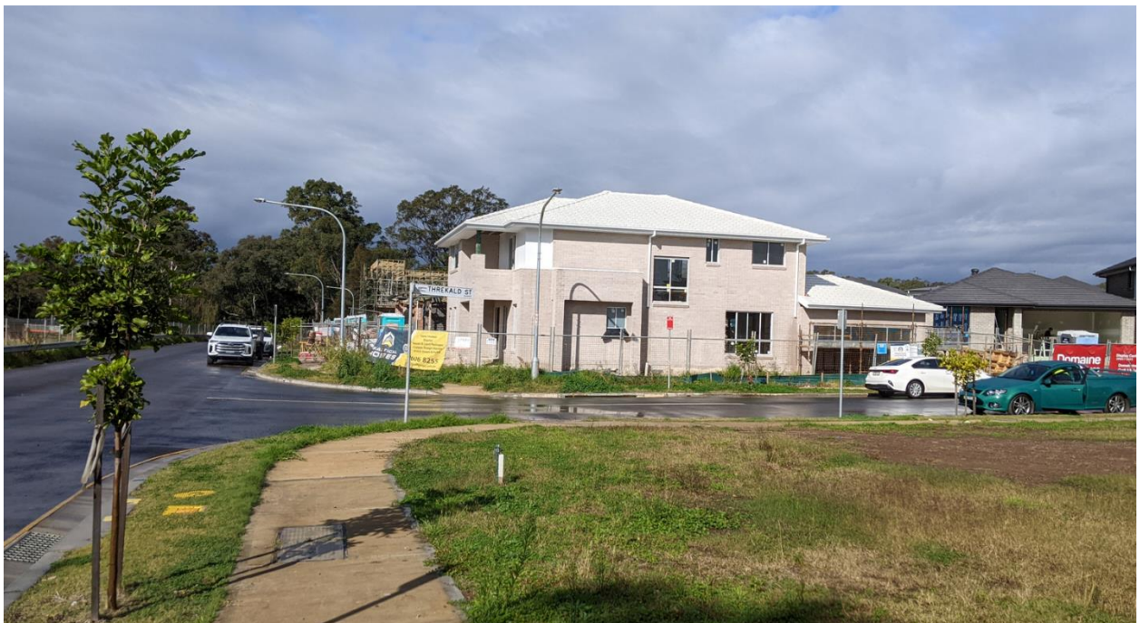
Figure 6 – View of recently/under constructed dwellings at 14 Flood Avenue (centre) and 4 Threlkald Street (right).
