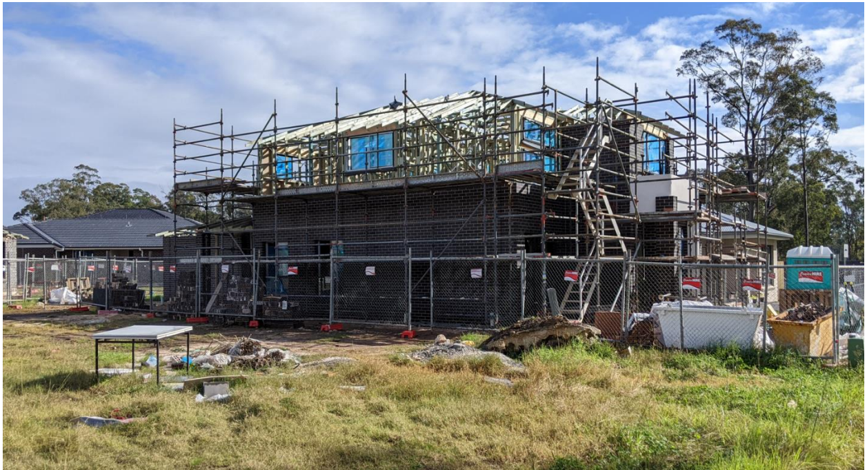
Figure 5 – Under construction dwelling on 20 Flood Avenue (two lots to the northwest).
