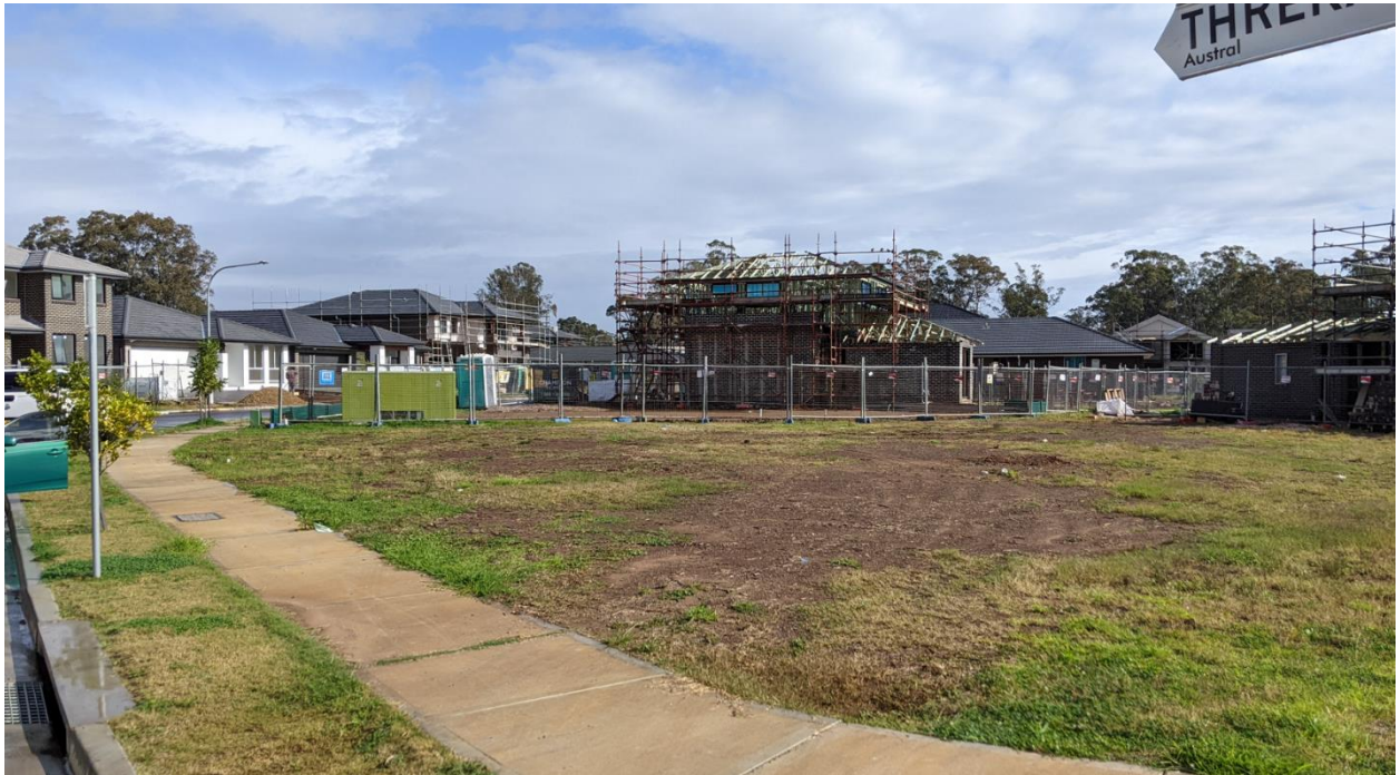
Figure 3 – Photo of the site at the corner of Flood Avenue and Threlkald Street, including the substation on 3 Threlkald Avenue.
