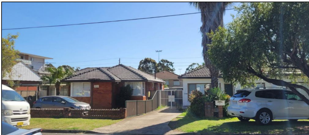
Figure 8: View of the western neighbouring dwelling on 23 Pearce Street
