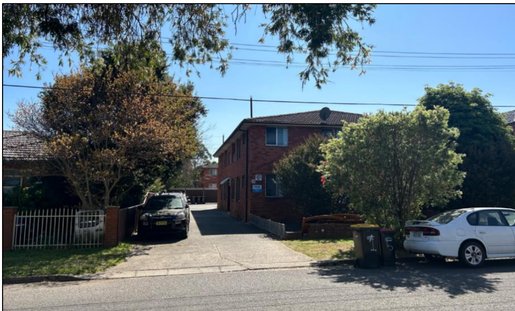
Figure 9: View of the eastern neighbouring two storey brick residential flat building on 13 Pearce Street
