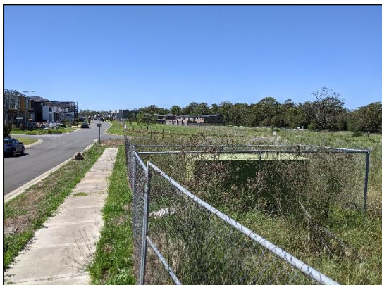
Figure 4: View east from Changsha Road, including the existing substation
