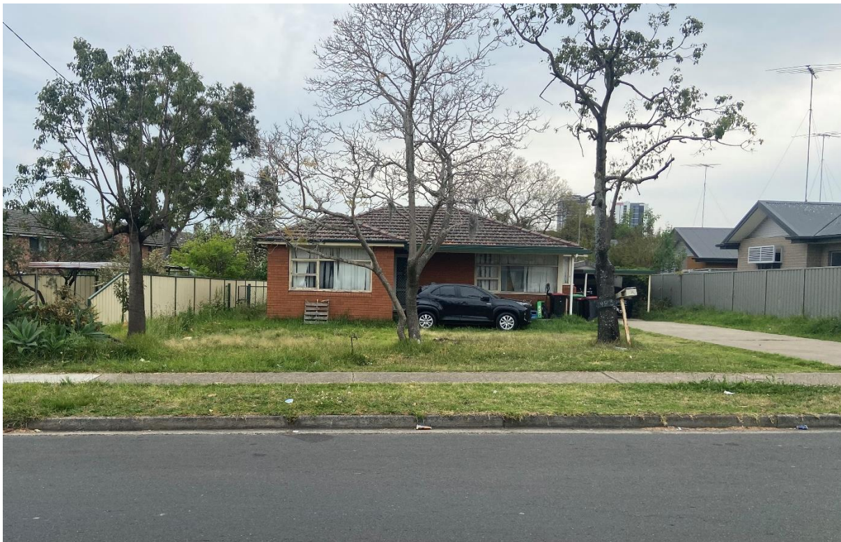
Figure 2: The existing dwelling at No. 3 Boundary Road.
