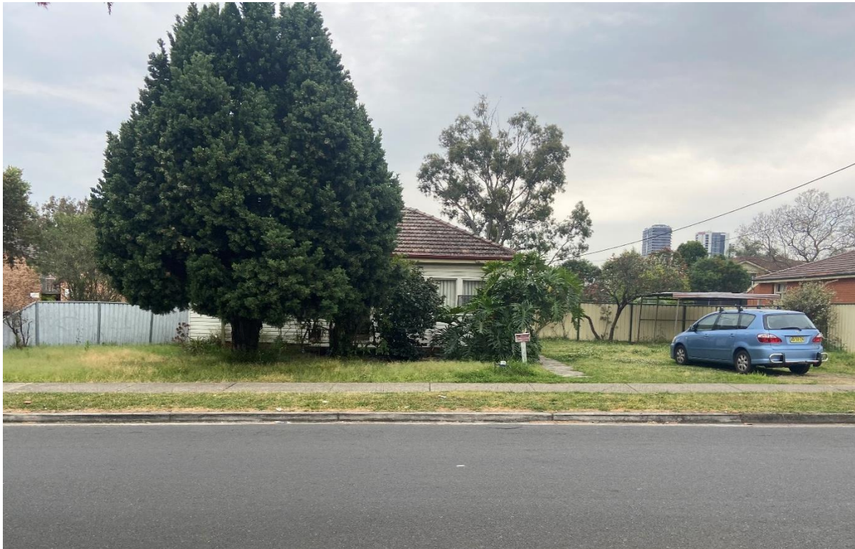
Figure 3: The existing dwelling at No.5 Boundary Road.
