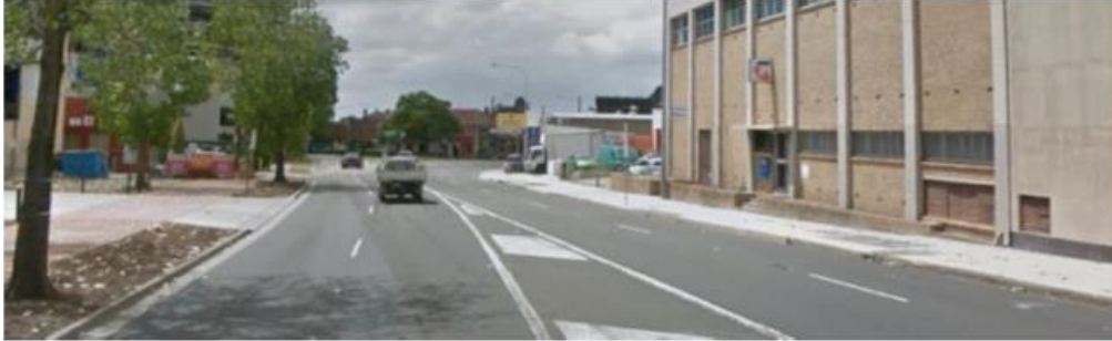
Source: Google map street view, Eastbound towards Newbridge Road
