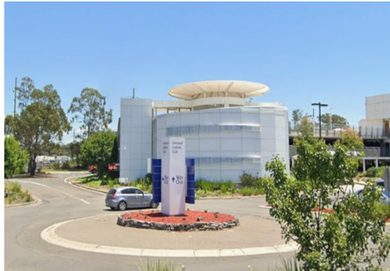
Figure 9: View of the multi-level car park and site entrance off Joadja Road looking west. (Source: Google Maps)
