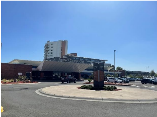
Figure 3: View of Liverpool Catholic Club from the central portion of the site facing north-east (Source: Keylan)
