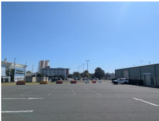
Figure 5: View of Liverpool Catholic Club, hotel, ice rink and car parking from southern portion of the site facing north (Source: Keylan)
