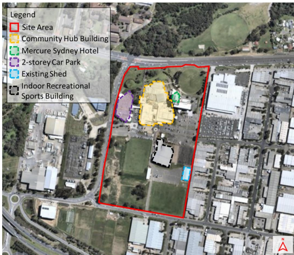
Figure 11: Existing improvements on the site (Base source: Nearmap)
