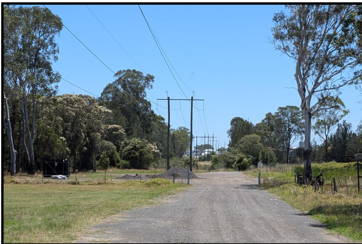
Figure 20: View north along the transmission easement at the eastern end of the site
