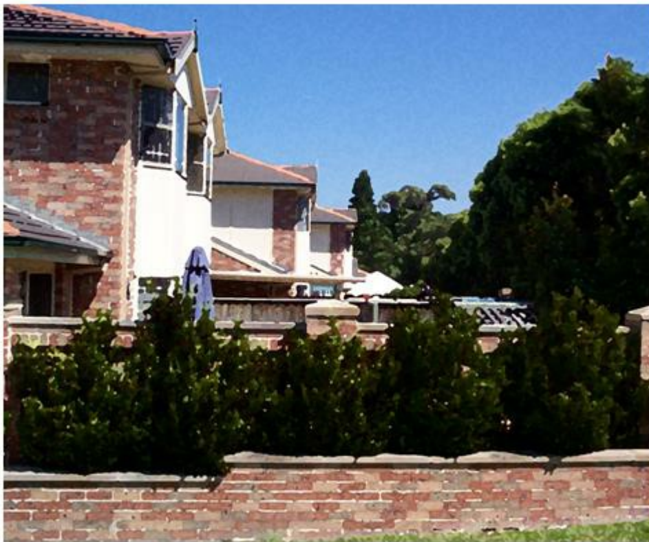
Figure 14 Fencing within Setback
