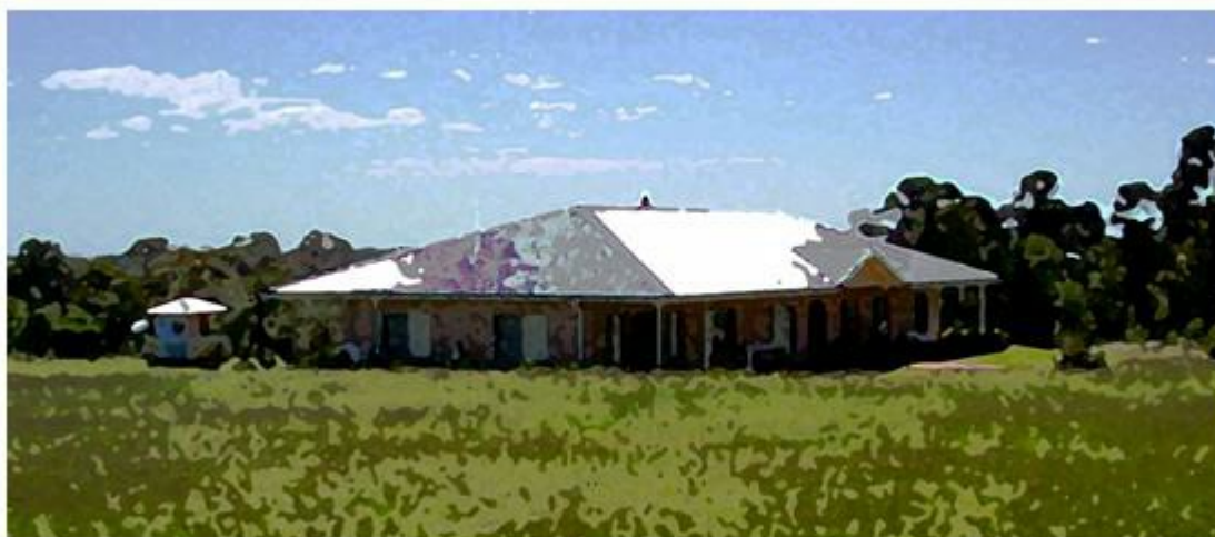
Figure 5 Poor Roof Design
