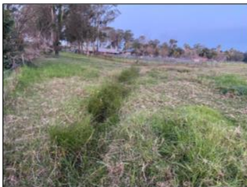
Figure 3.4 View northeast across the northern section of the project area showing an excavated drainage channel
