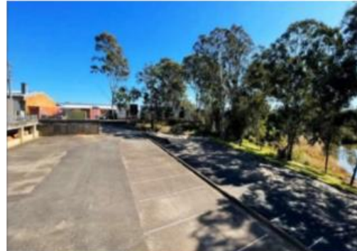
Figure 6 View of part of the rear lower portion of the site and carpark showing part of the banks of Lake Moore
