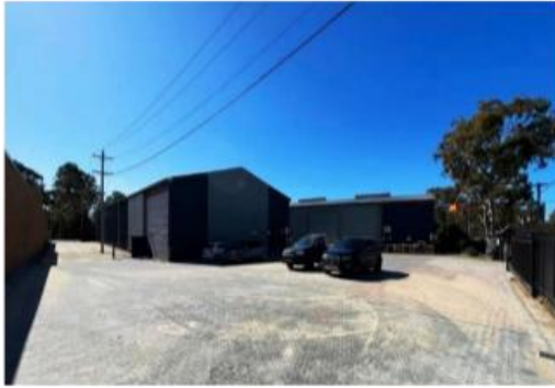
Figure 5 View of part of the front portion of the site and front loading area
